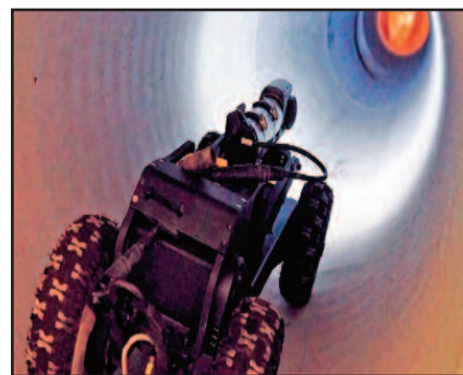
Crawler cameras are remotely-controlled, self-propelling, and able to record high-quality videos and images of sewers and pipelines. The camera's transmitter sends signals above ground that provide information about the direction of the pipeline, as well as the exact location of potential problem areas.
