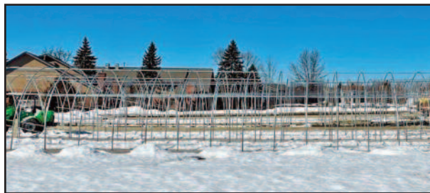
Quonset huts now under construction at Platt Hill
