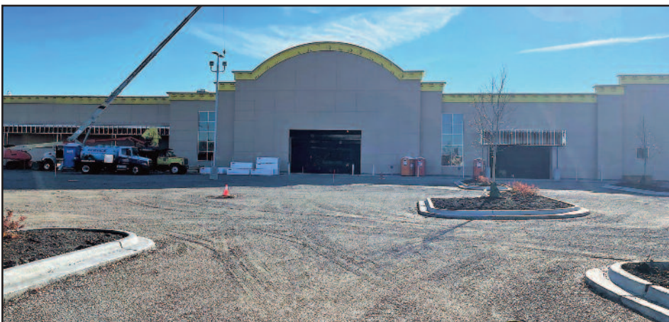
The roof is now on!
